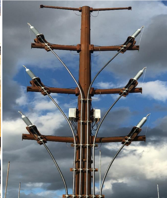
Right: All 6 terminations are complete at the Hershey Sub.
