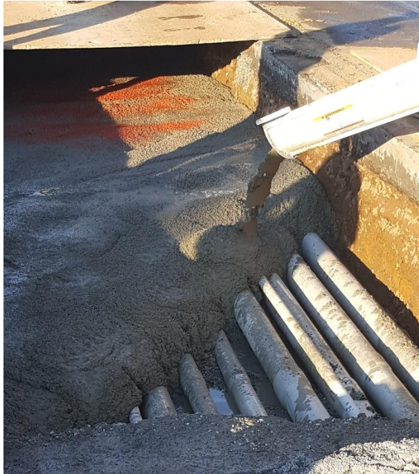
Left: Final conduit installation on Sand Hill Rd.
